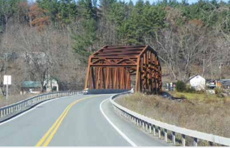
Truss Köprü (Schoharie Creek - NY/USA)
